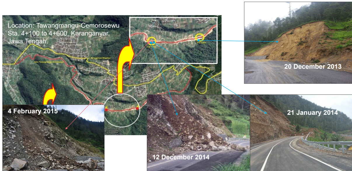
Figure 7: Debris deposit of the roadside slope failure: Tawangmangu-Cemorosewu road in Central Java
