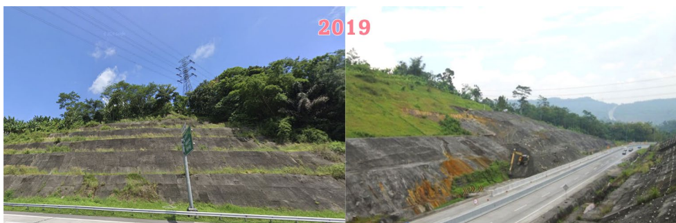
Figure 9: Slope remedial measures using shotcrete and bolt at Toll Road Semarang-Bawen: (left) successful work, (right) unsuccessful work
